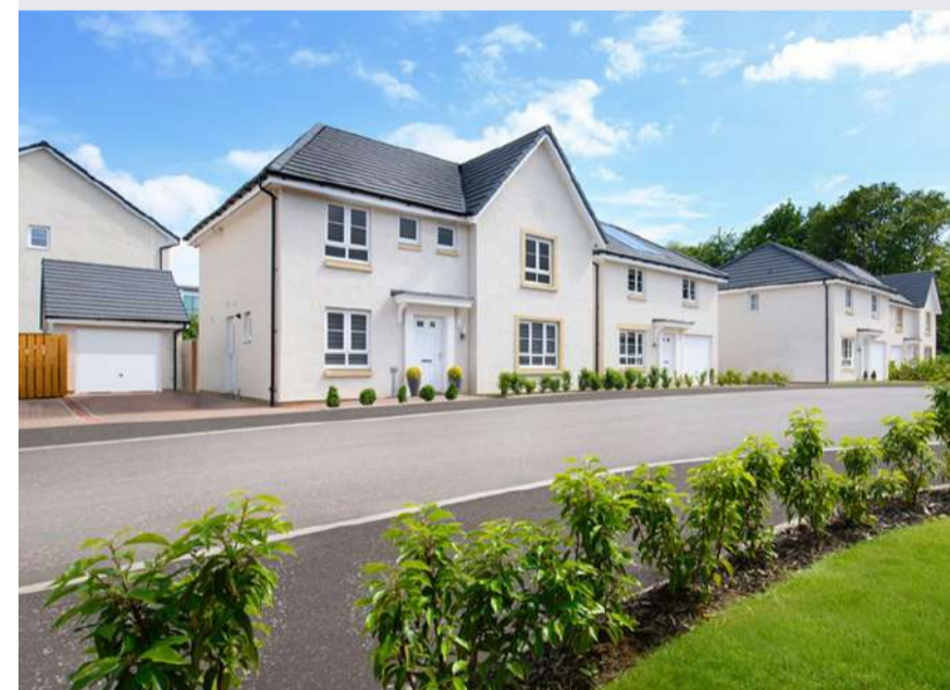
BARRATT HOMES - Thornton View, 228 new homes approved on the western outskirts of East Kilbride
