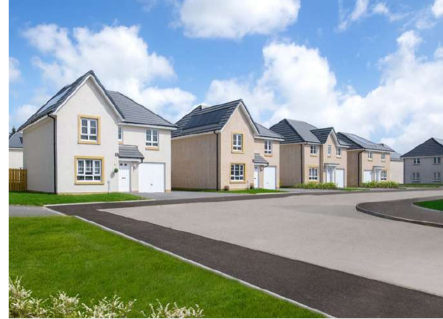
BARRATT HOMES - Merlin Gardens housing development, 315 new homes adjacent to the application site's eastern boundary, currently under construction
